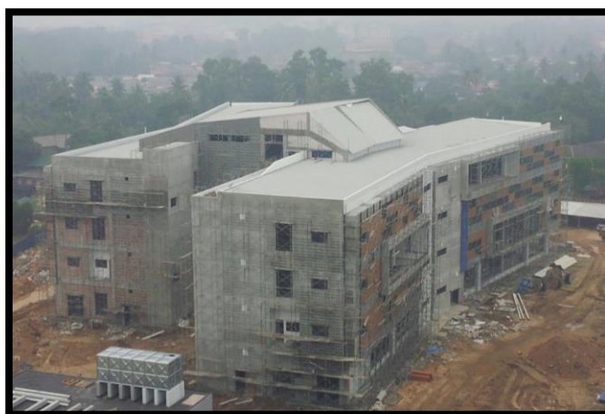
Figure 1: PPAP building construction process
